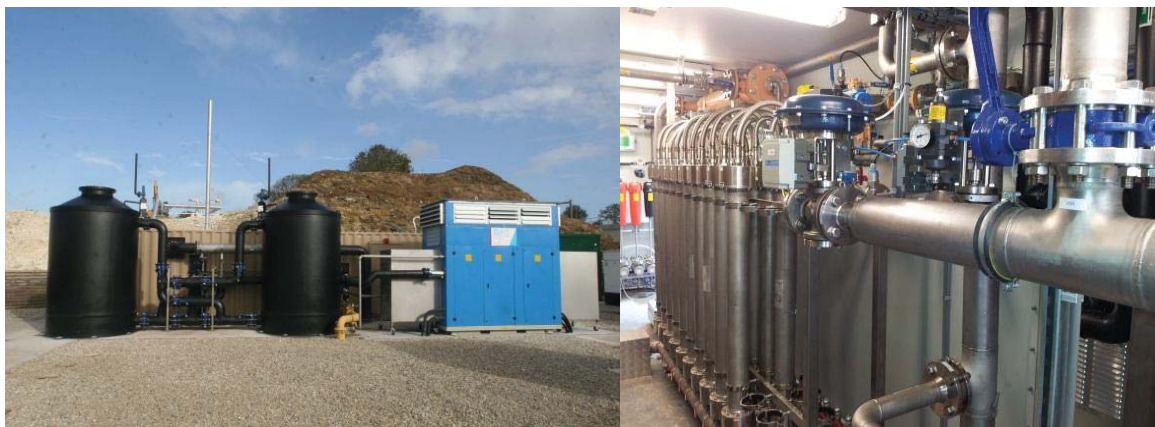
Figure 16 The membrane biogas upgrading plant in Poundbury with a capacity of 650 Nm 3 /h raw biogas. Images from DMT.
