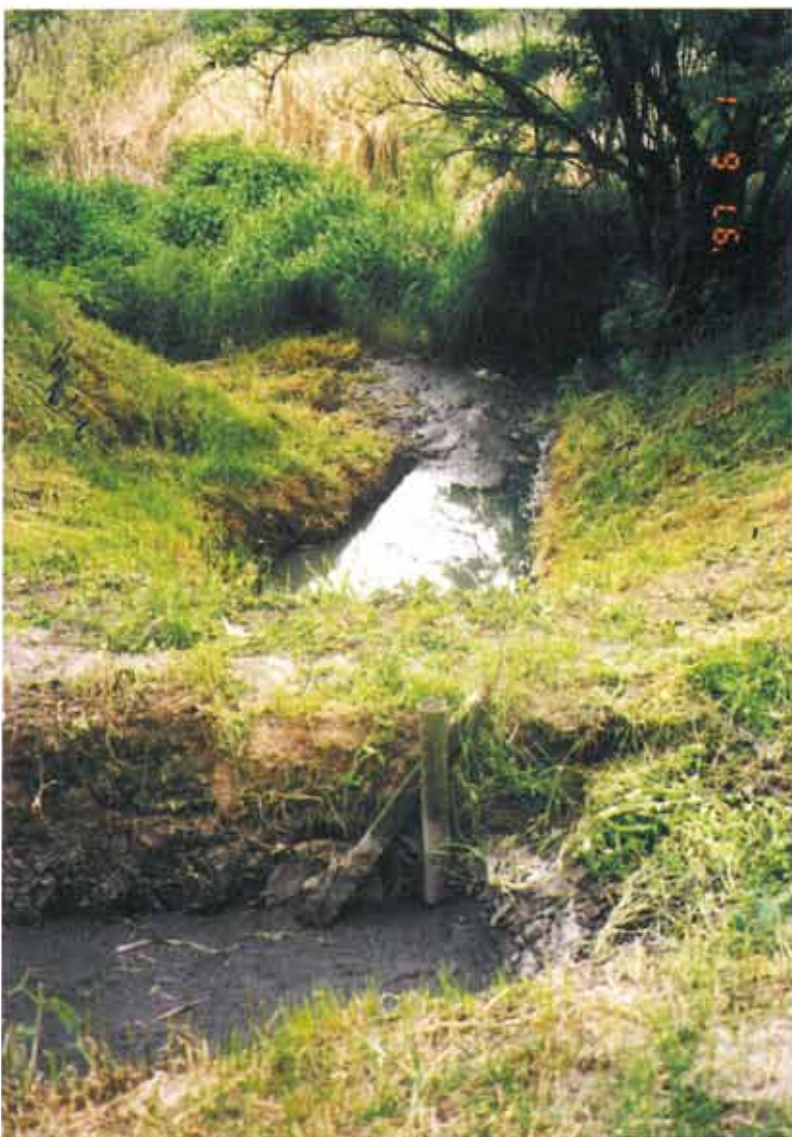
Figur A5. Infiltrationsdamm i bruk, Wansdorf
